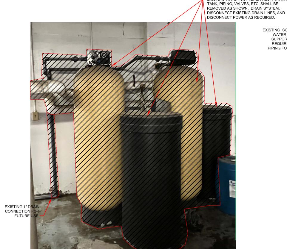
DOMESTIC WATER PUMPS TO REMAIN. SUPPORT EXISTING PIPING AS -EXISTING WATER SOFTENER RESIN TANK, BRINE REQUIRED. MODIFY EXISTING PIPING FOR TIE-IN TO NEW PIPE.—
