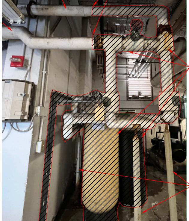
EXISTING WATER PIPING, VALVES, SUPPORTS, ETC. SHALL BE REMOVED AS SHOWN.
